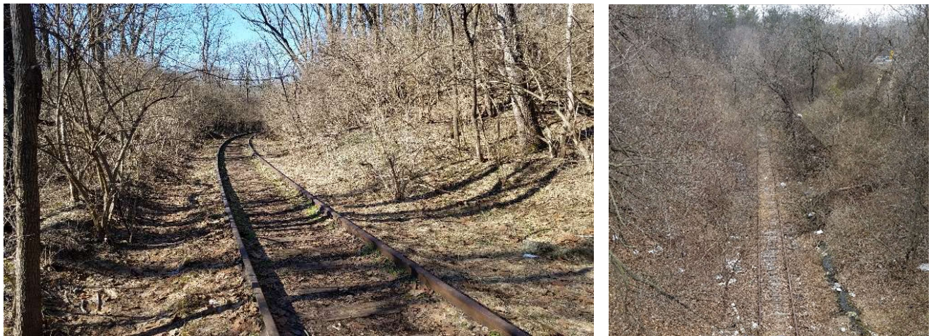
Figure 1a – A Future Trail? Rail line noted as Future Martin Tower Spur Trail on map above. On left, viewed from Monocacy Way Trail. On right, viewed from 8 th Avenue.
