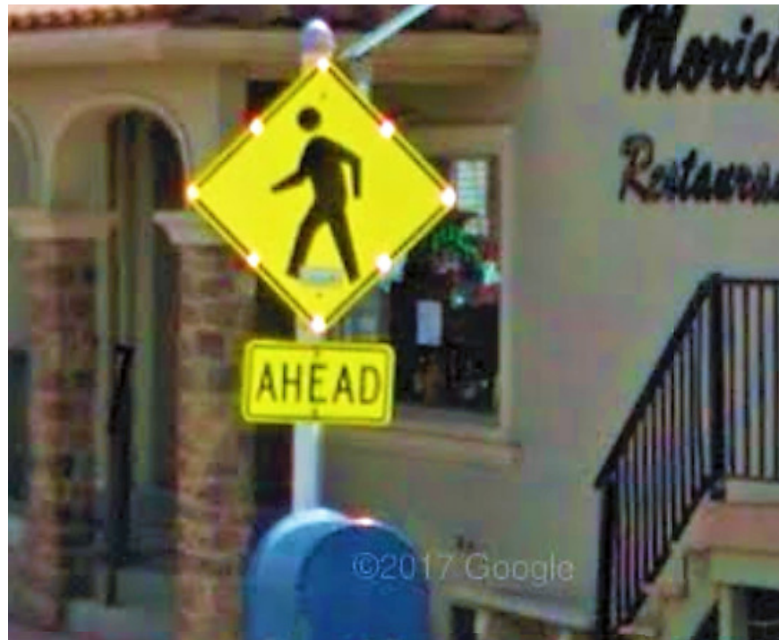
Figure 7 – Existing pedestrian “Ahead” flashing lights on Cattell St. (solar) are not push button activated and could be relocated to a crosswalk and used with push-button activation
