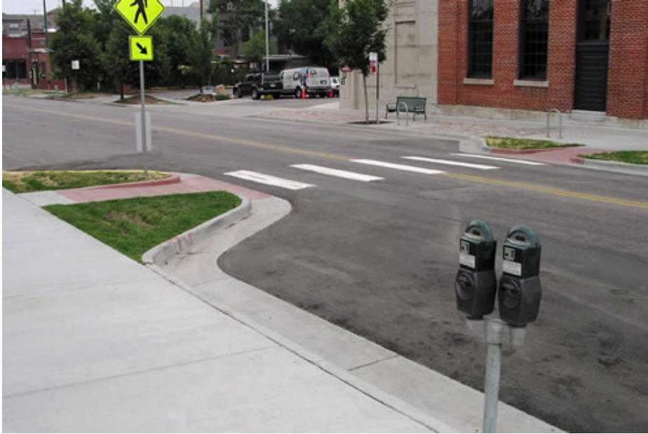
Figure 5 – Pedestrian curb extensions and painted high-visibility crosswalks
