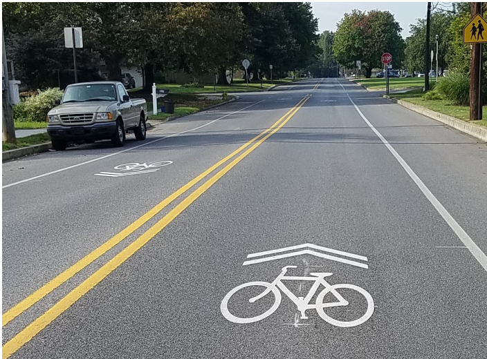
Figure 10 – Bicycle Shared Lane Marking
