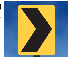
Figure 14 – W1-9 Chevron Warning Signs
