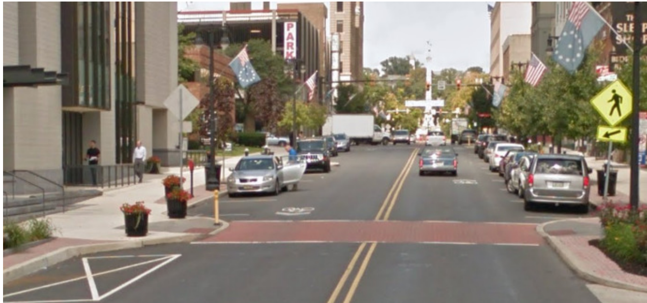
Figure 6 – Pedestrian curb extensions and high-visibility faux-brick inlay crosswalks
